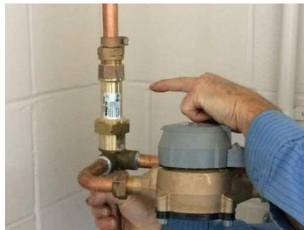
All water connections installed after 1972 are required to have a check valve as part of the meter installation. Older connections without check valves are upgraded to the new standard when the meter setting is changed or upgraded. Eventually all connections will have some sort of backflow preventer.
